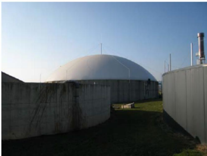
Image 12: Biogas plant/fermentation tank with foil gas storage
